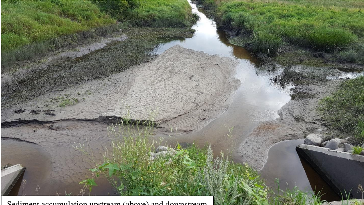
Sediment accumulation upstream (above) and downstream (below) of the CSAH 54 crossing of the Moose River
