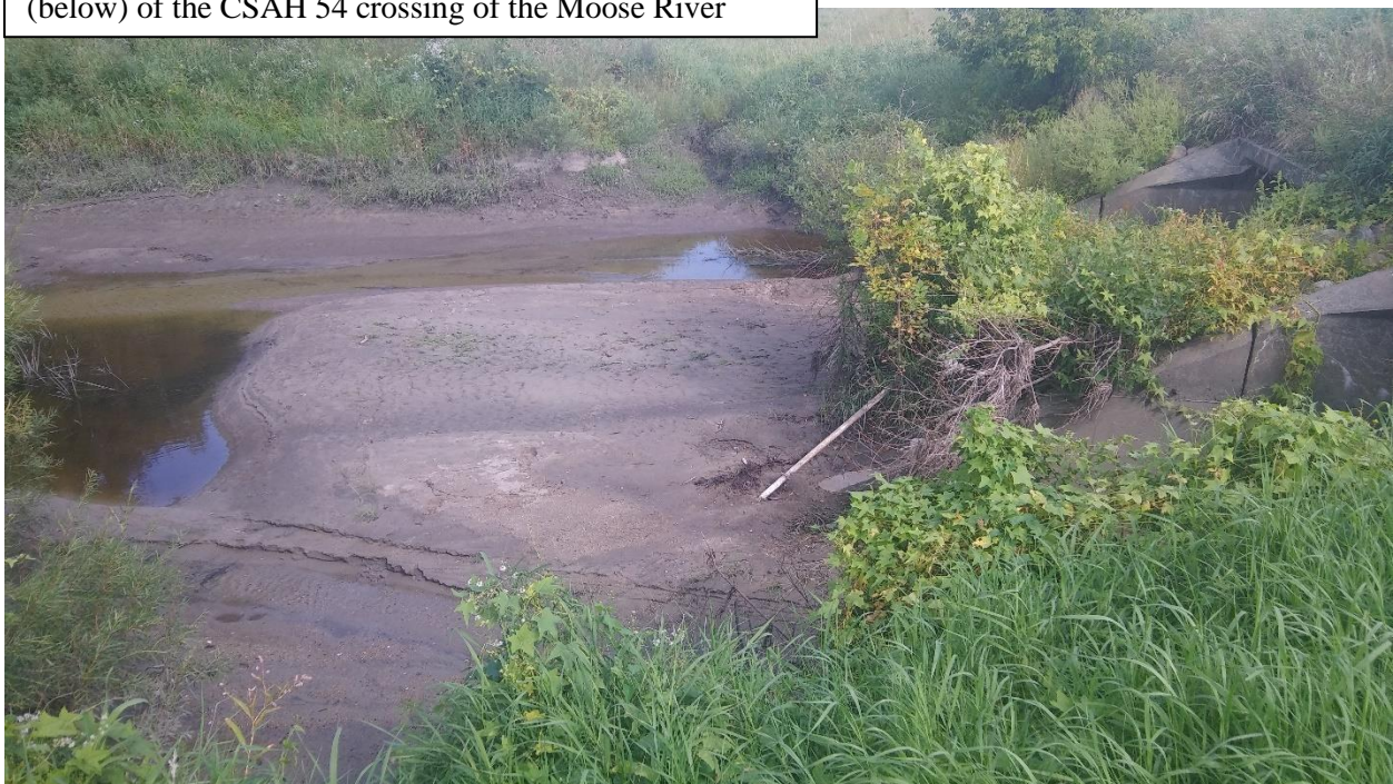
Sediment accumulation upstream (above) and downstream (below) of the CSAH 54 crossing of the Moose River
